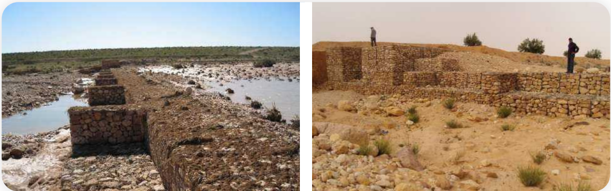
Figure 15 Gabion Check Dams
