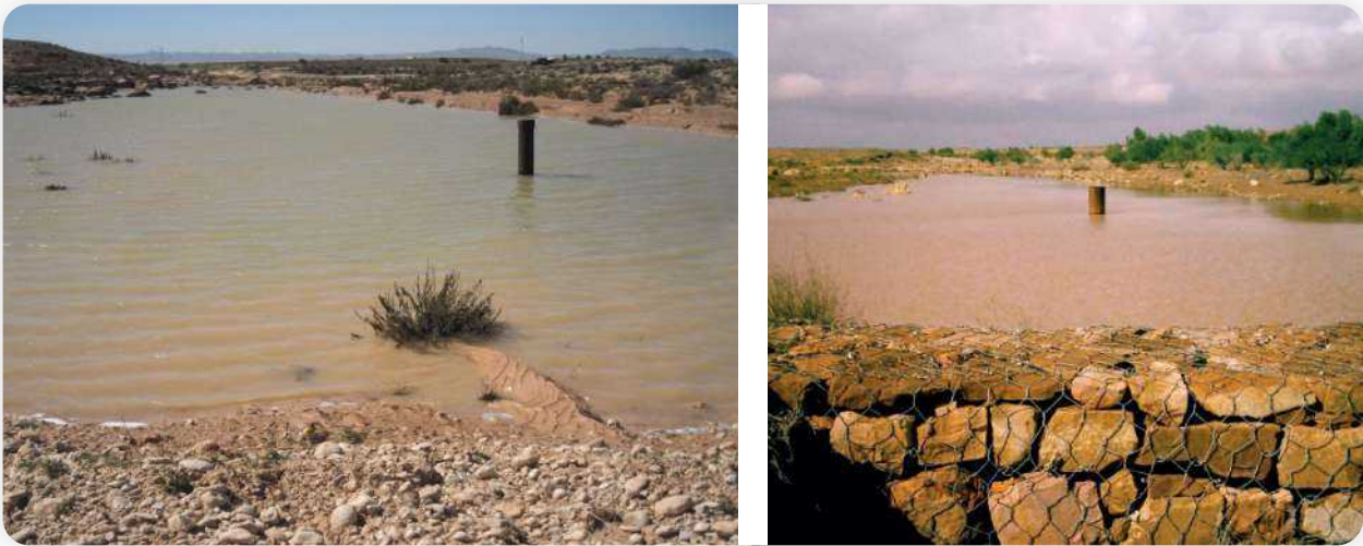
Figure 24 Recharge Well behind a Gabion Check Dam
