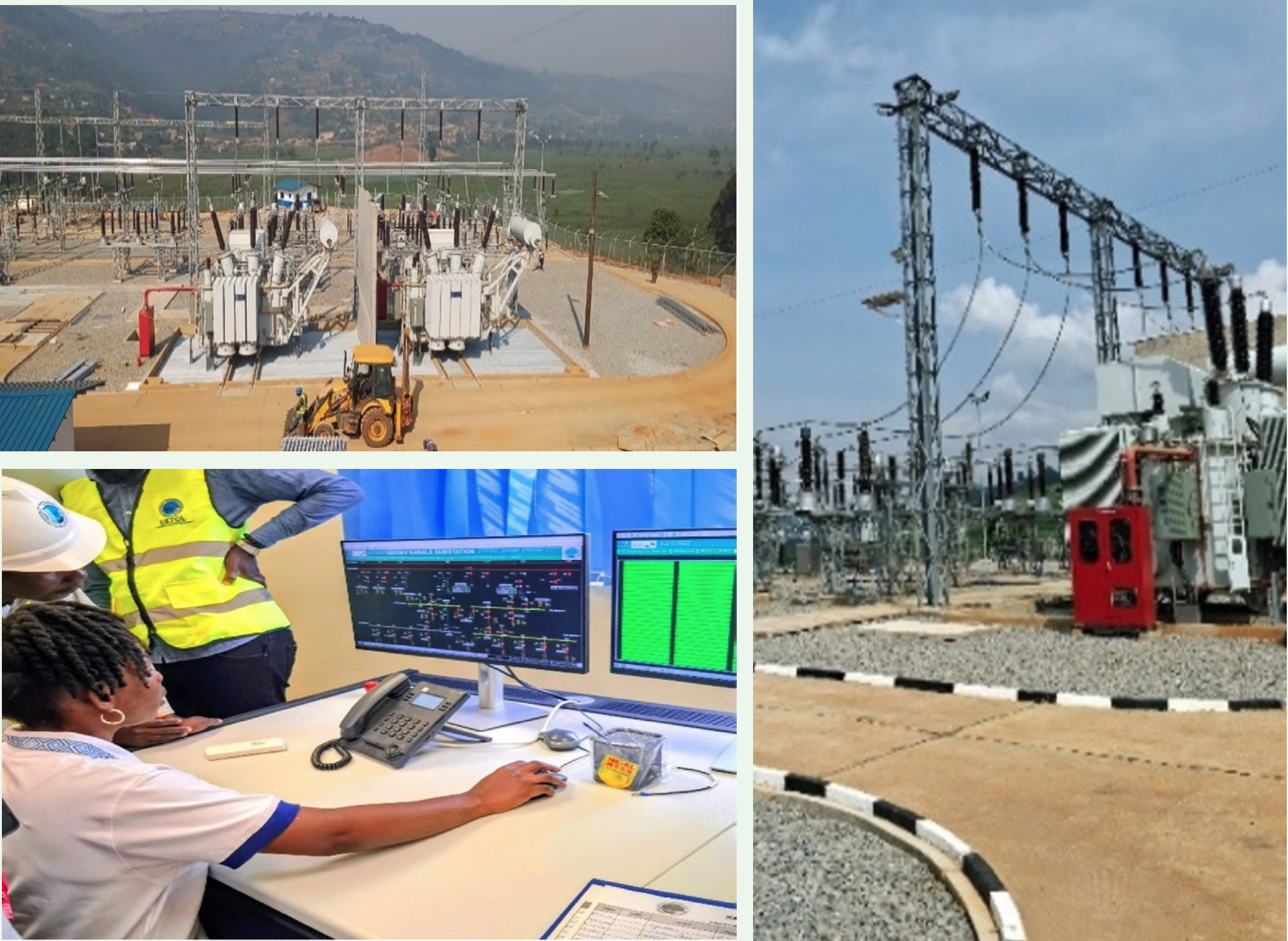
Photo 2: Mirama–Kabale Transmission Line and Distribution Project (Uganda)
