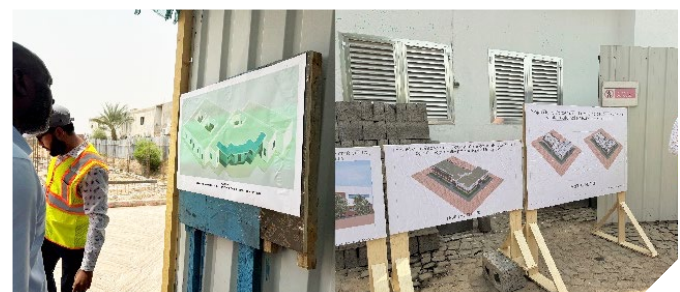
Hospital under construction/renovation
