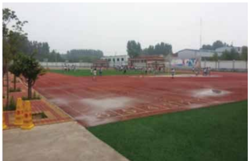
RENOVATED SPORTS FACILITIES IN AN IDB-SUPPORTED SCHOOL IN CHINA
