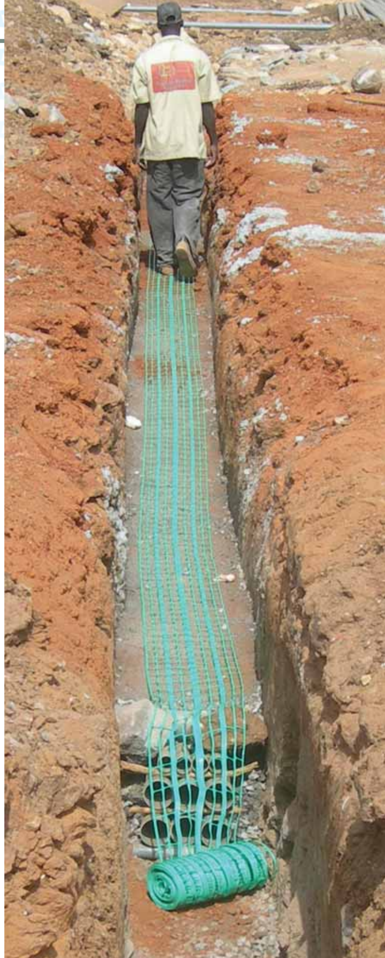
PHONE NETWORK RELOCATION FOR UPGRADING OF DAKAR EXPRESSWAY
