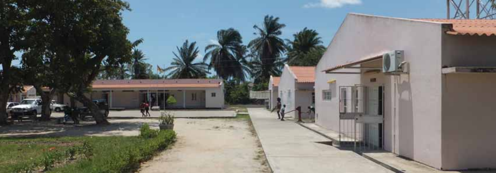
RENOVATED SCHOOL IN MOZAMBIQUE
