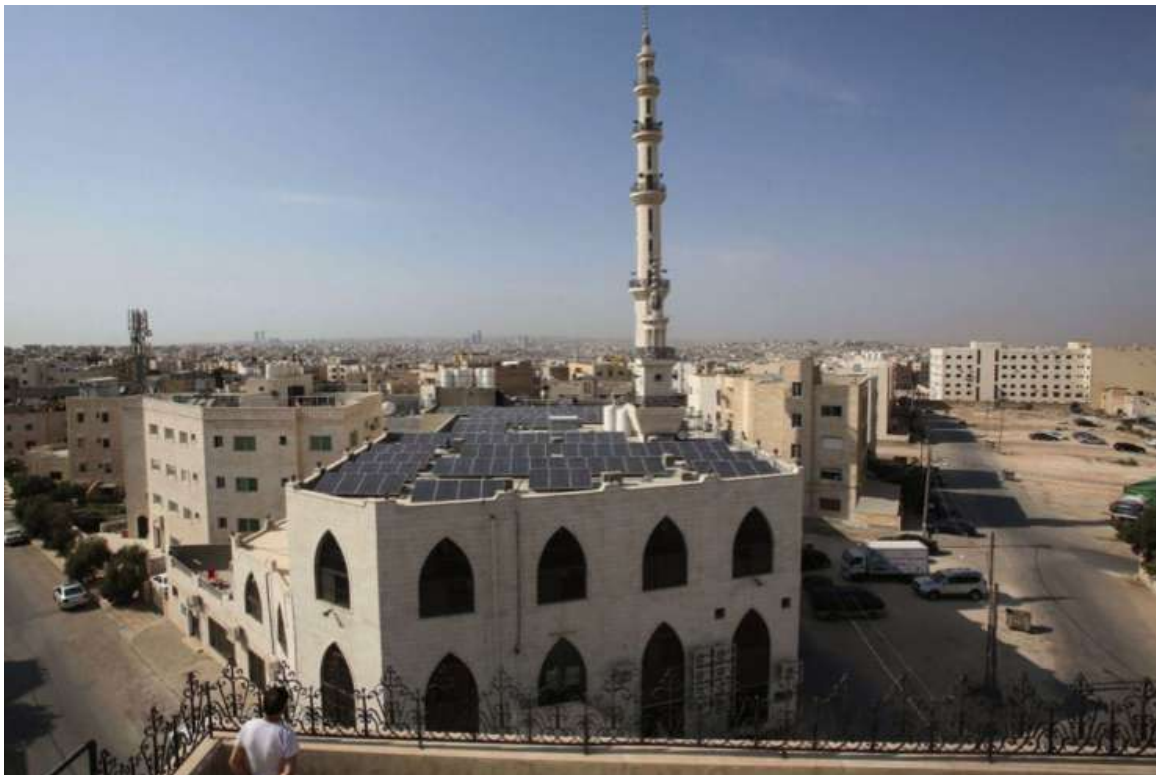
Figure 4.6: The Hamdan al-Qara mosque in southern Amman covered in rooftop PV panels
