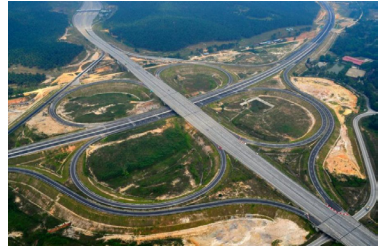
Figure 1: 33km LATAR Expressway in Malaysia; Co-financed by IsDB
