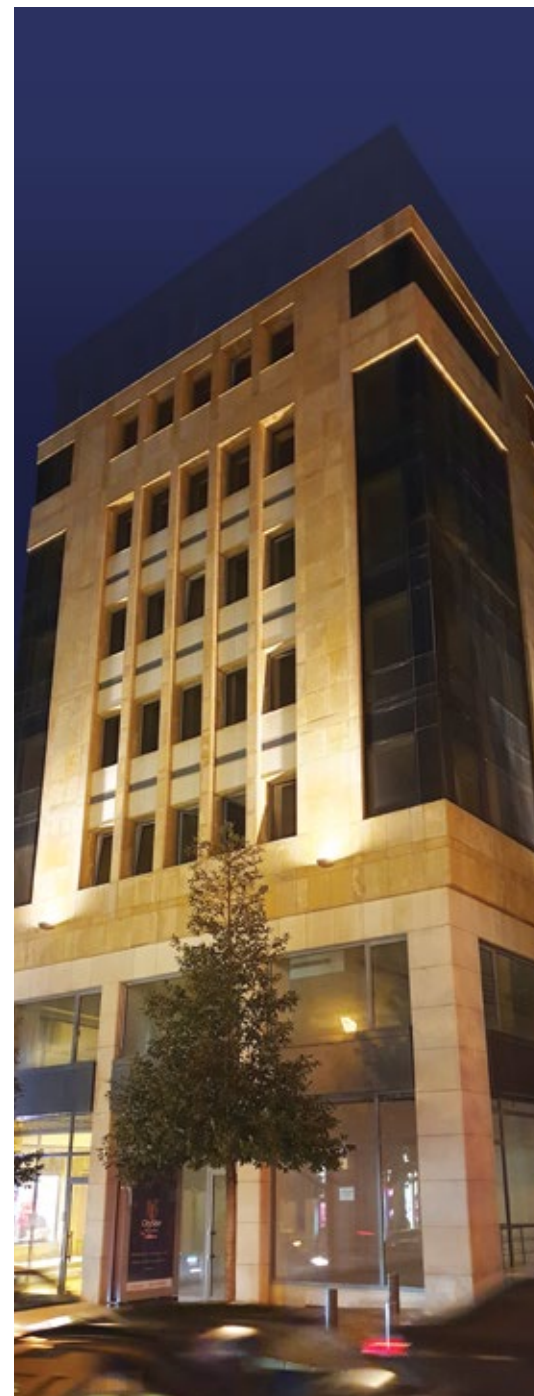
Makassed Philanthropic Islamic Association, Beyrouth, Liban Projet Bazerkan Building Waqf. Source: FIBA
