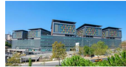
IsDB-funded Okmeydani Training & Research Hospital
