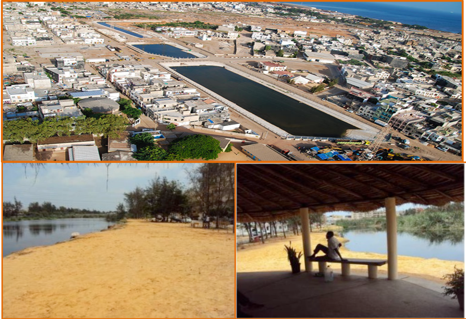
Photo 3: Installation of Balancing Ponds to Attenuate Peak Rainfall Events
