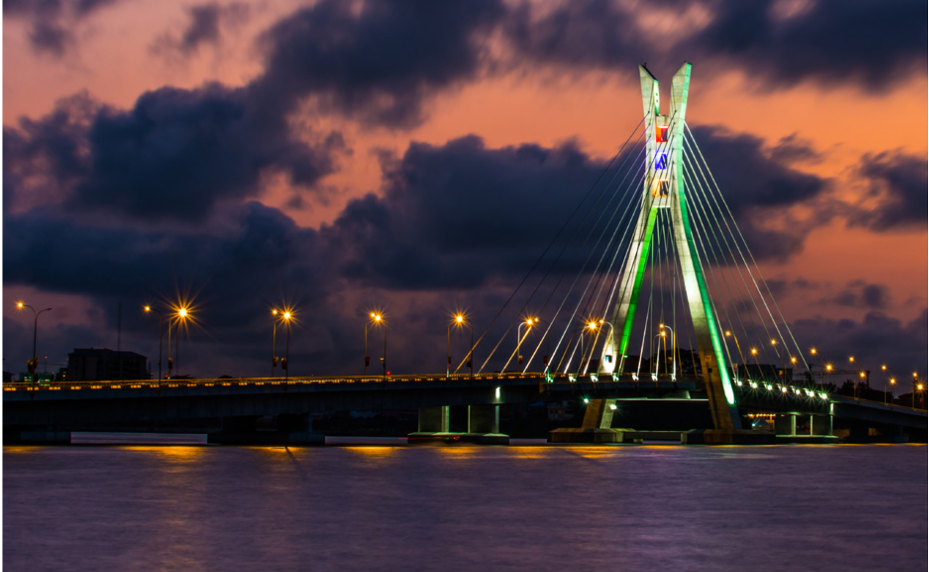
The Lekki-Ikoyi bridge, Nigeria. New technologies, such as big data and the Internet of Things, are widely used in new infrastructure projects and have made it easier to connect the developers of various infrastructure assets to their users, with the effect of increasing the capacity to manage more sustainable infrastructure projects
