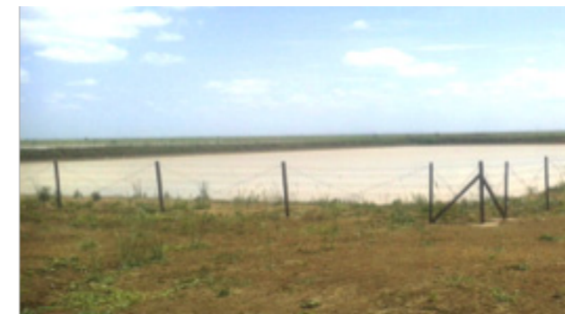
Figure-6: Small water dam pond of the Water Harvesting Project for Agro-Pastoral Development in Al- Gadarif State of Sudan
