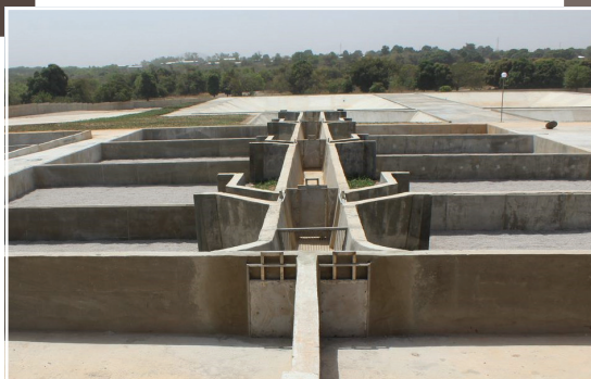
Model sludge treatment plant that will be replicated in the cities covered by this project
