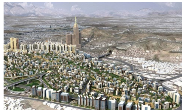
Figure 2c Jabal Alsharashif new master plan Source: Al Balad Al Amin Company, http://albaladalameen.com.sa/ab/arproject.php?mid=49&msid=34#
