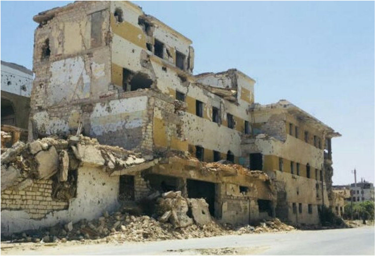
Destroyed building in Benghazi, Libya. June 2018. Photo: Alex Koclejda/NRC
