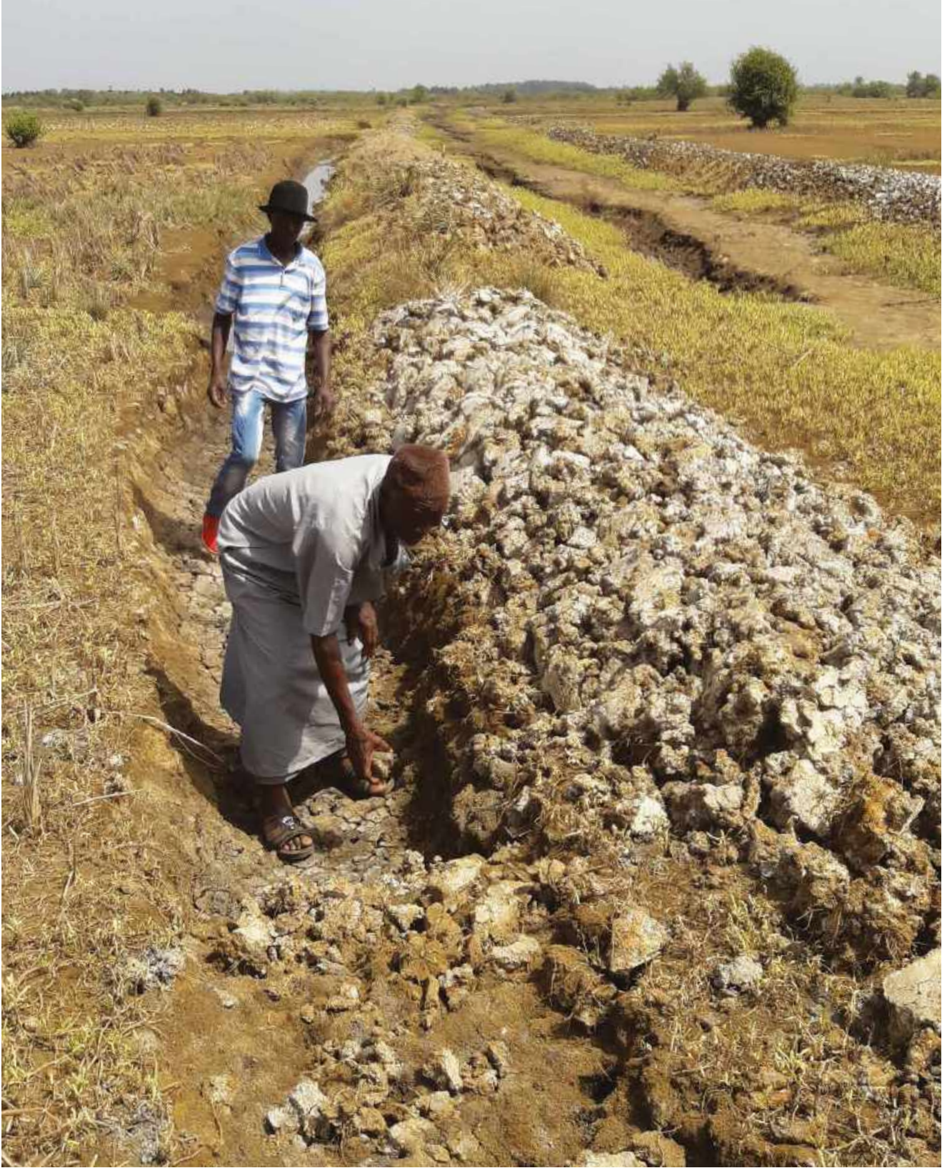
Smallholders in Guinea maintain bunds to control flooding from the sea. Floods create saline soils that are difficult to grow crops in.
