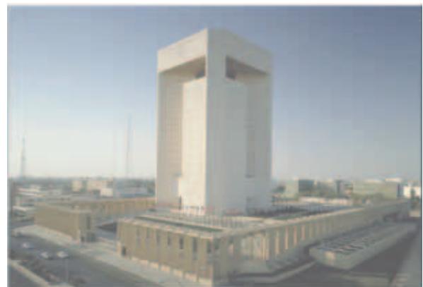
IDB Headquarters in Jeddah, the Kingdom of Saudi Arabia
