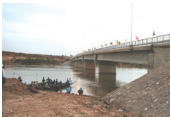
The IDB extended a loan of an amount of ID9.3 million ($12.2 million) for the construction of the Gao Bridge in Mali. The bridge was completed in September 2006 and is expected to link the Trans Saharan Road to the national road network as well as roads coming from neighbouring member countries, i.e. Niger and Burkina Faso.
