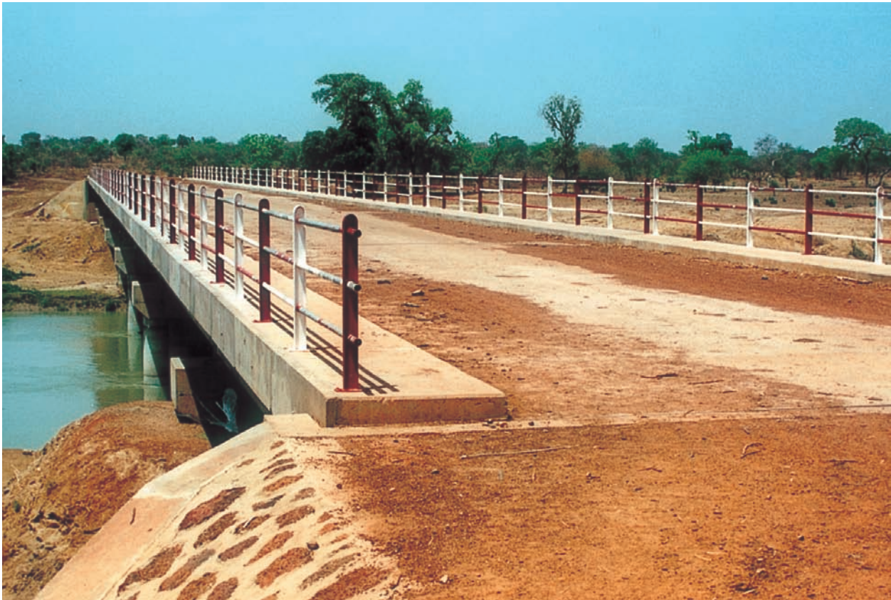
Development of Rural Infrastructure is a key area of IDB financing
